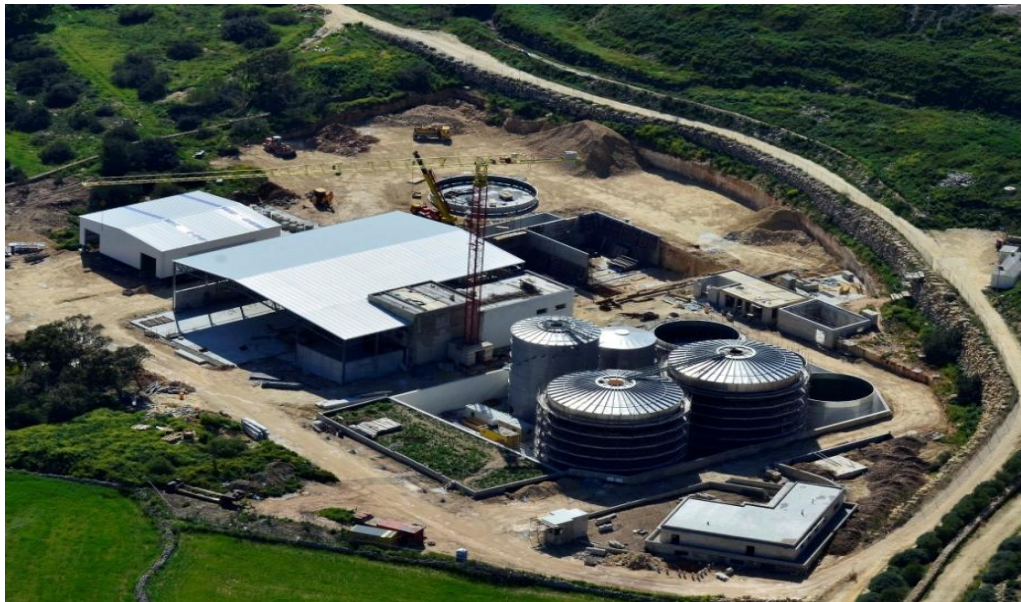
Malta North Treatment Facility - Aerial Photo of Project Site
