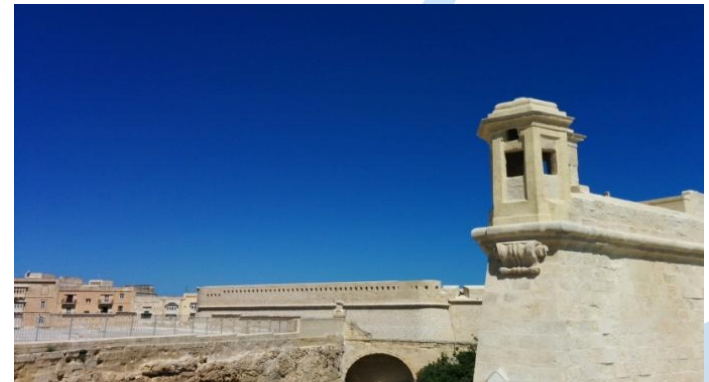
ERDF244 – Restoration of St Elmo Bastions
