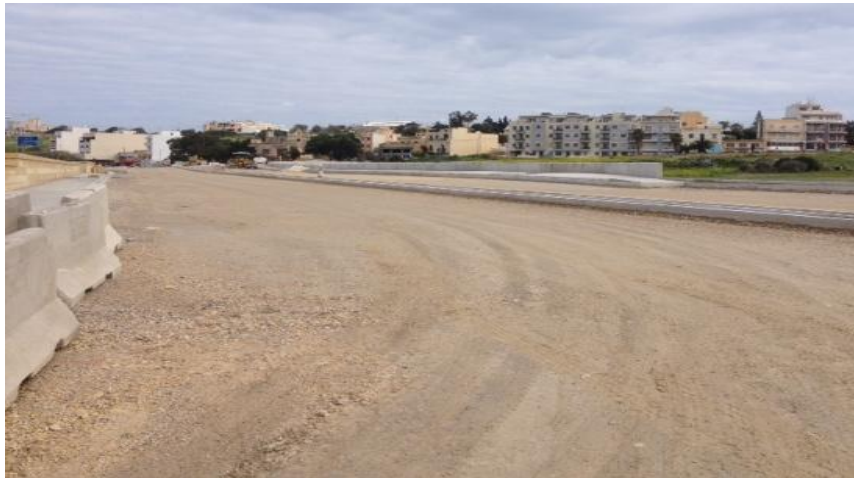
Phase 2: Road Works leading to the Bugibba Junction
