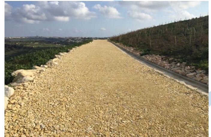
Rehabilitation of Qortin landfill - Upper access road and storm-water gutter
