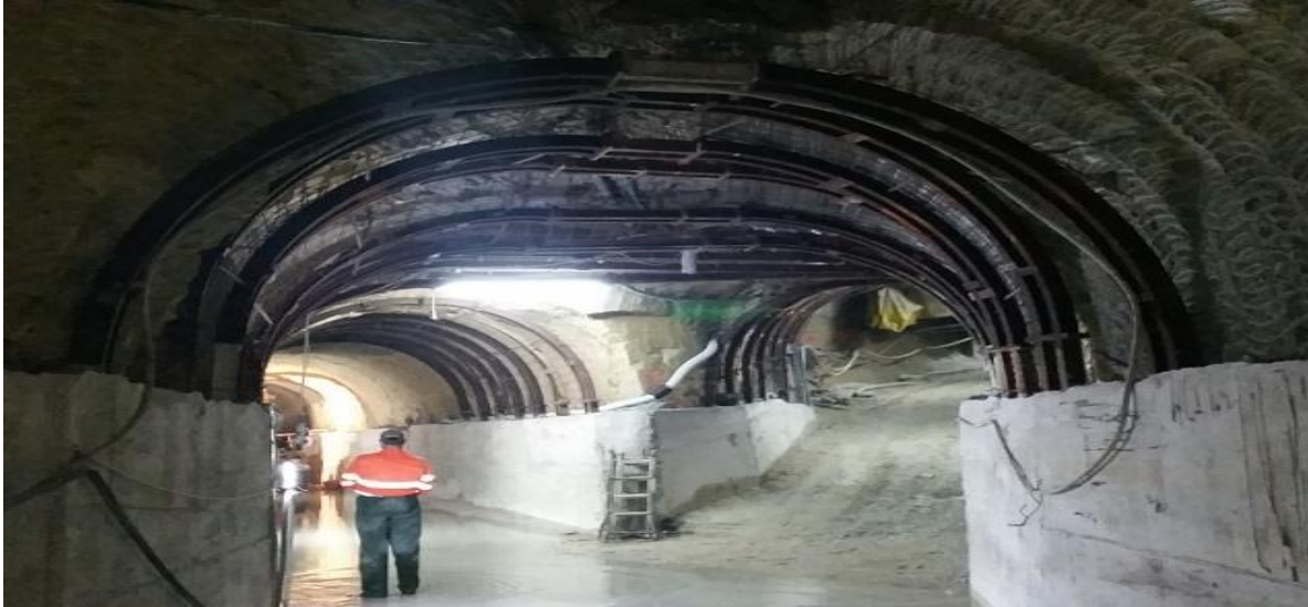
NFRP - Zabbar Tunnel
